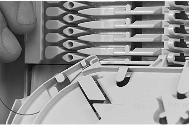
4.3.7 Pull gently on the fibers in the tray and make sure that the fibers are well contained in FAS block and wraparound groove plate.
