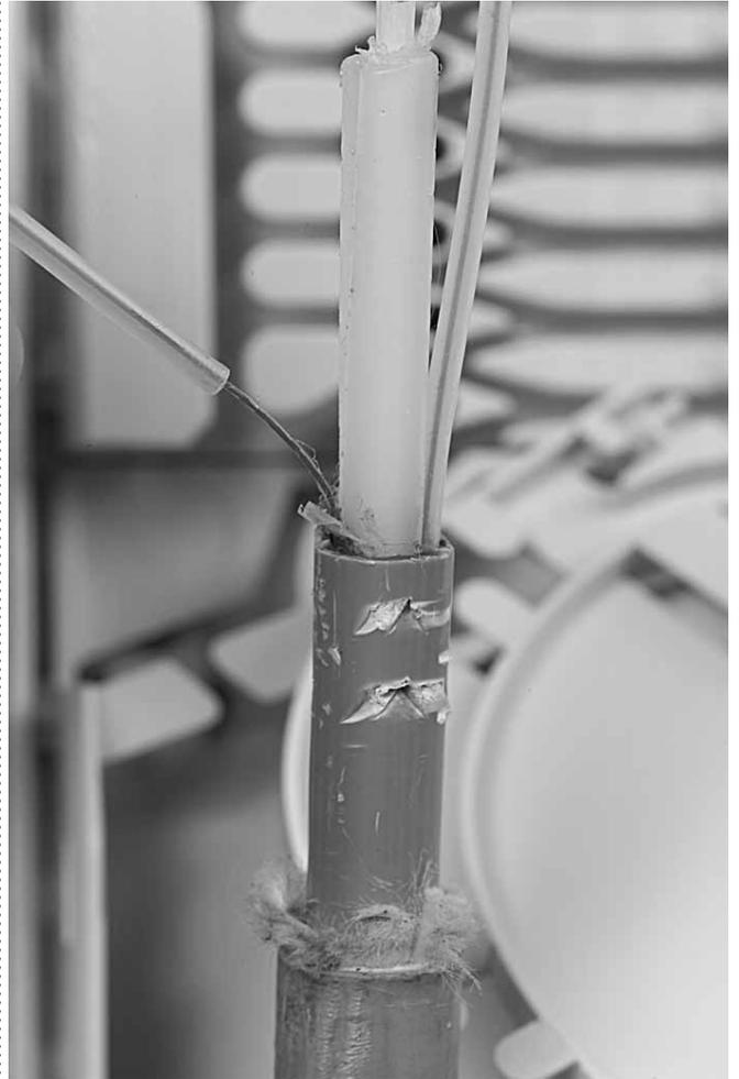
4.1.3.1 Install a protection tube of 150 mm over the fibers of each slot and slide it into the slot of the cable.
