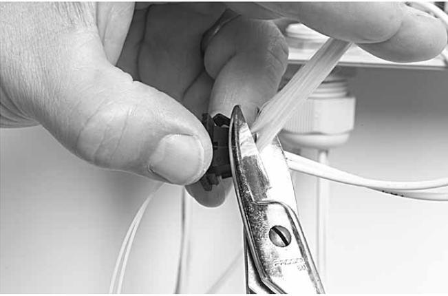
5.2.8 Cut the Kevlar yarns at the connector and install in the patch panel adapter.
