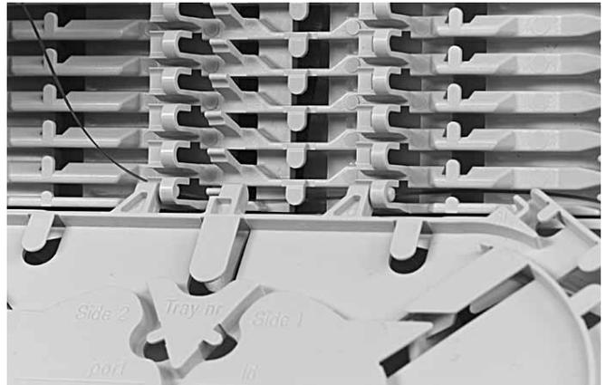
4.3.6 Route the fibers in the grooves of the wraparound groove plate to the entrance of the identified tray. Fiber must be routed in the groove of the tray hinge.
