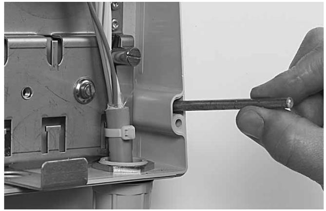
7.5 In case of a box with lock insert first the four guiding pins in the box before installing the cover.
