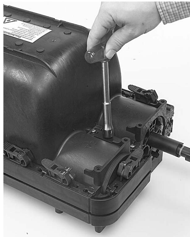
3.8.5 Use a nut driver to tighten the captured bolt at each end of the closure.
