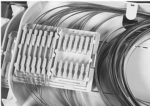
3.5.20 On the tray there's the possibility to store the splices in two different compartments (top and bottom). The first completed splices have to be stored in the bottom compartment, in the splice holders farthest from the hinge. When all bottom slots are full, the top slots can be filled.
