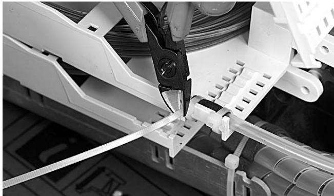
3.5.6 Mark the FOPT at 15 mm on the tray and remove the tube excess. Secure the FOPT with 2 tie-wraps and trim the tails.
